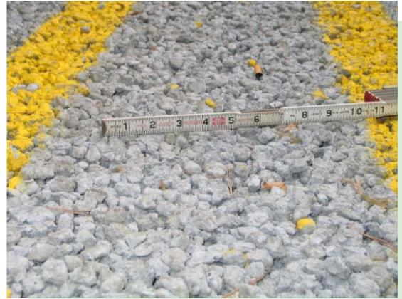
***Filtered naturally ...*** Pervious concrete pavement helps filter water runoff and reduces the strain on wastewater treatment facilities.
